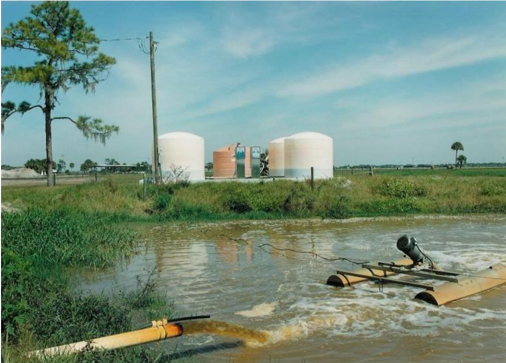
This is the bioreactor for a large Florida dairy farm barn and pasture runoff treatment system that used metallic salts addition for enhanced phosphorus control.
